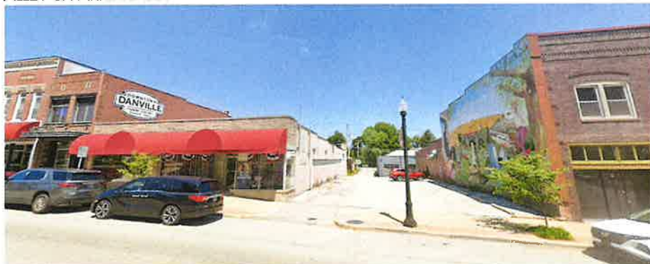
ADJACENT BUILDING TO WEST, ACROSS ALLEY
