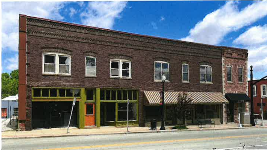
EXISTING FRONT/SOUTH ELEVATION W/ADJACENT BUILDINGS TO EAST
