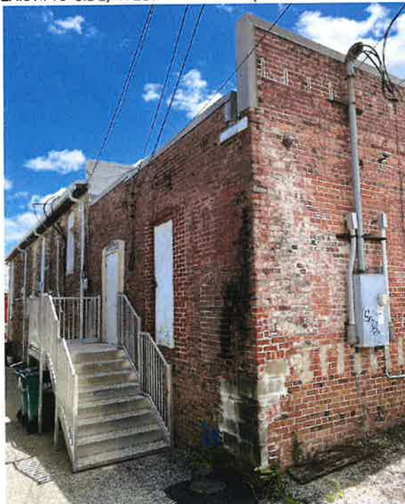
EXISTING REAR/NORTH ELEVATION IN PEDESTRIAN ALLEY
