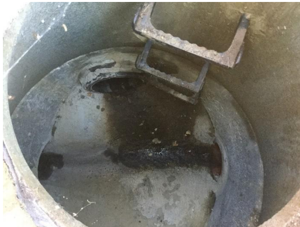
Sanitary Manhole. Top of photo is North.
