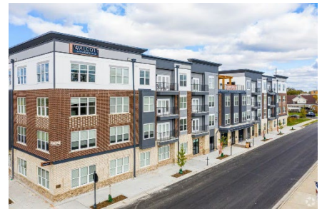
Example of Flat Roof
